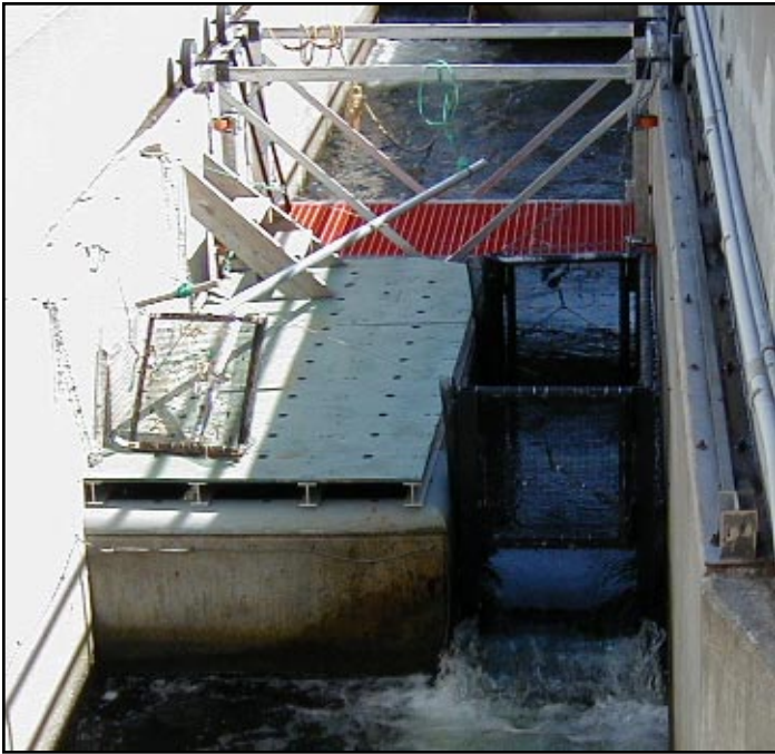
View looking east taken from the patio above Ballard Locks fish viewing chamber. The fish trap used to capture native steelhead is shown positioned in the weirs. --Photo by Fred Zingleman
